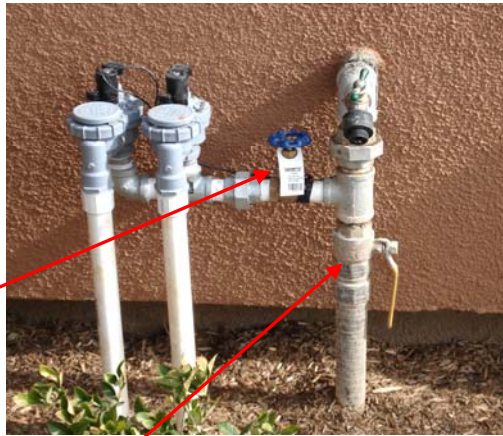
House Valve or Gate Valve
